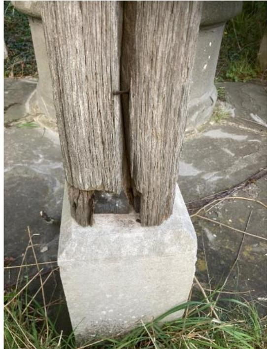
Part of the foot of one timber post has broken away, as shown in the photograph.
